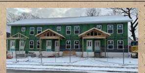
For the building located at 32-34 Munsell (pictured above), the exterior and interior walls have been constructed, the roof is 90% completed, the building is about 65% sided, all windows and doors have been installed and the interior has begun to be sheet fully plumbed and has been completely wired for electric.
